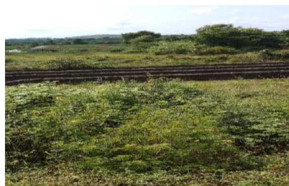
Barrel wall of partly constructed (1987) sluice
